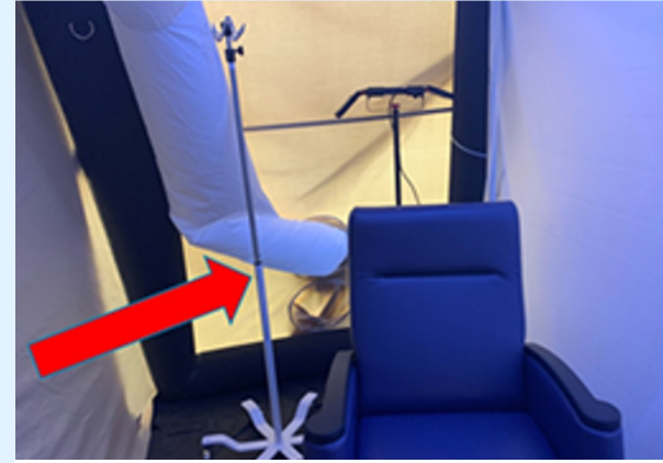
Bottom opening exhausted to create front to back airflow across patient
